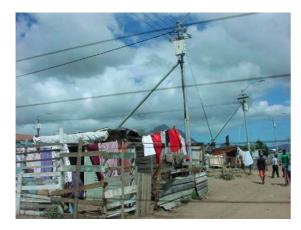
Fig. 2 Highly visible "maypole" type distribution system in Khayelitsha, Cape Town, South Africa makes electricity service drops less susceptible to theft [5]
