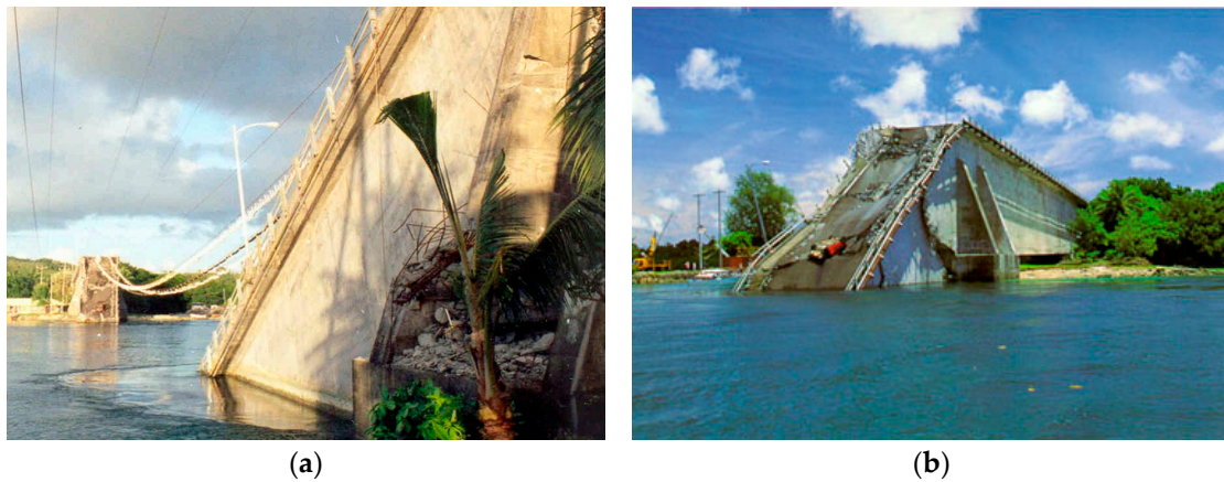
Figure 5. (a,b) The Koror-Babeldaob Bridge collapse [11].
