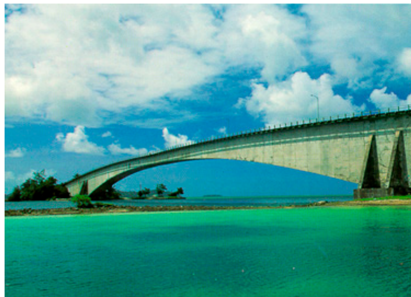
Figure 4. The Koror-Babeldaob Bridge, sagging of the middle point [10].
