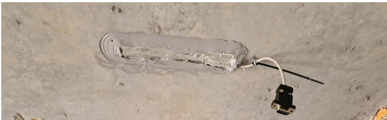
Figure 50. Strain gauge after protection
