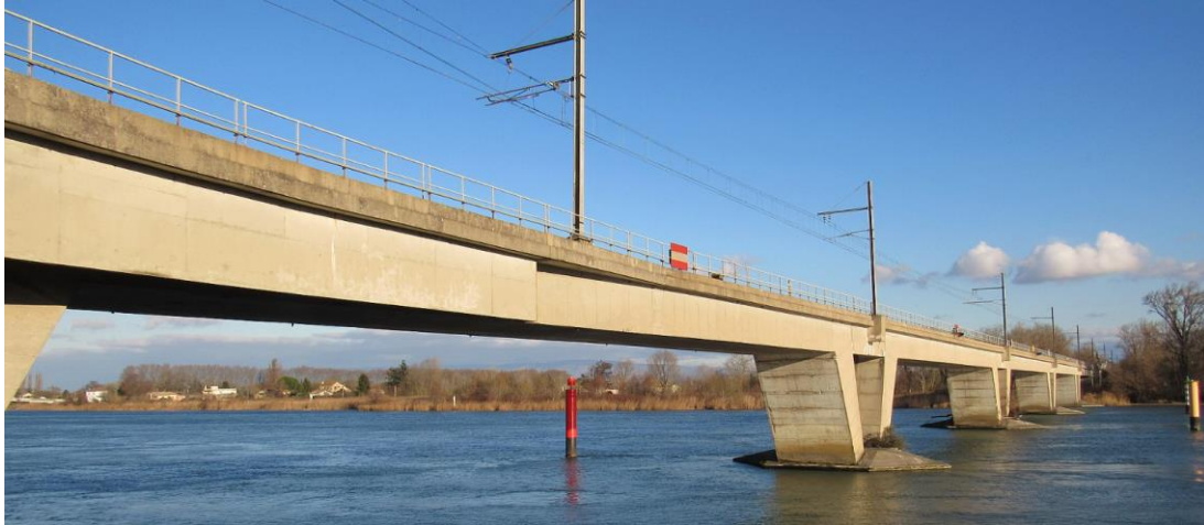
Figure 12. La Voulte railway bridge
