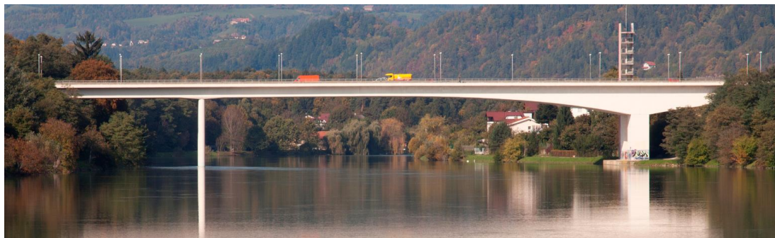
Figure 22. Carinthia Bridge in Maribor
