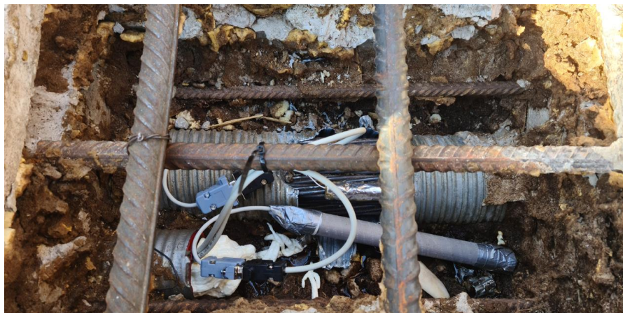
Figure 51. Strain gauge installation on prestressing cables (with temperature compensation)
