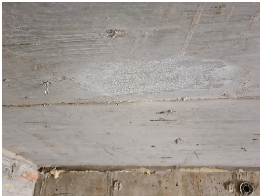
Figure 48. Surface prepared for gauge installation
