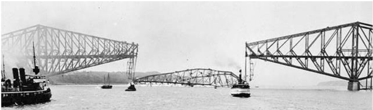
Figure 19. Quebec bridge, collapse of the central segment
