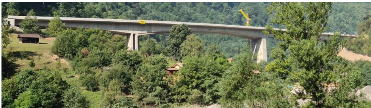
Figure 34. Vranduk 1 left and right bridge
