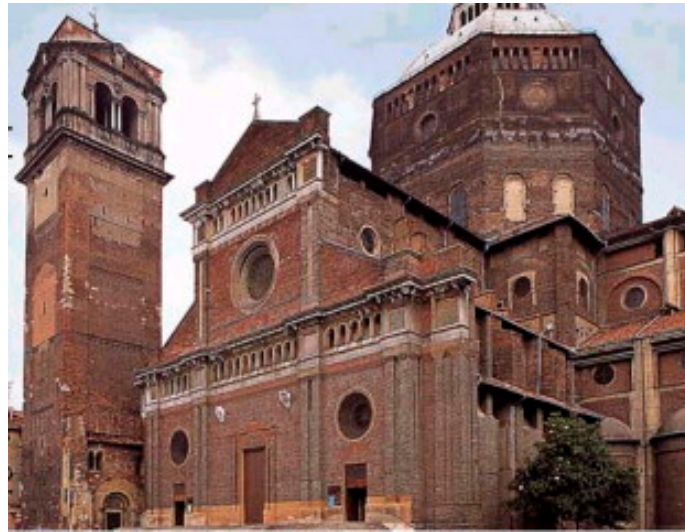
Figure 2. Civic Tower in Pavia, Italy, before the collapse [6].
