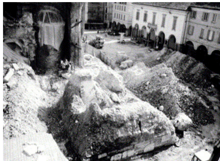
Figure 3. Remains of the Civic Tower in Pavia after the collapse [8].
