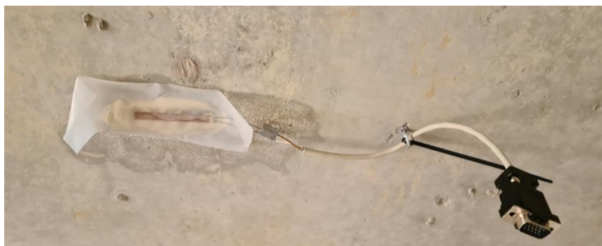
Figure 49. Installed gauge with the adapter after glue hardening
