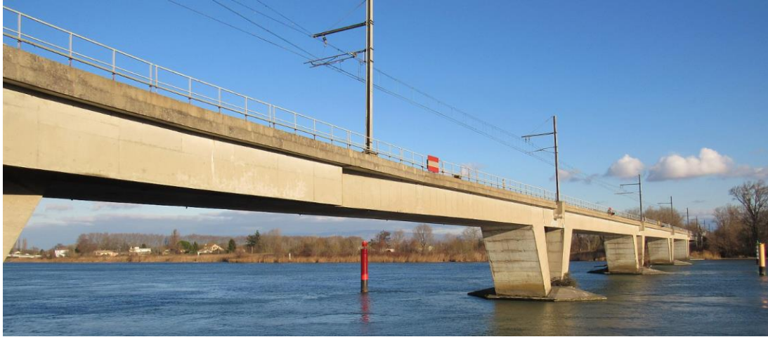
Figure 12. La Voulte railway bridge
