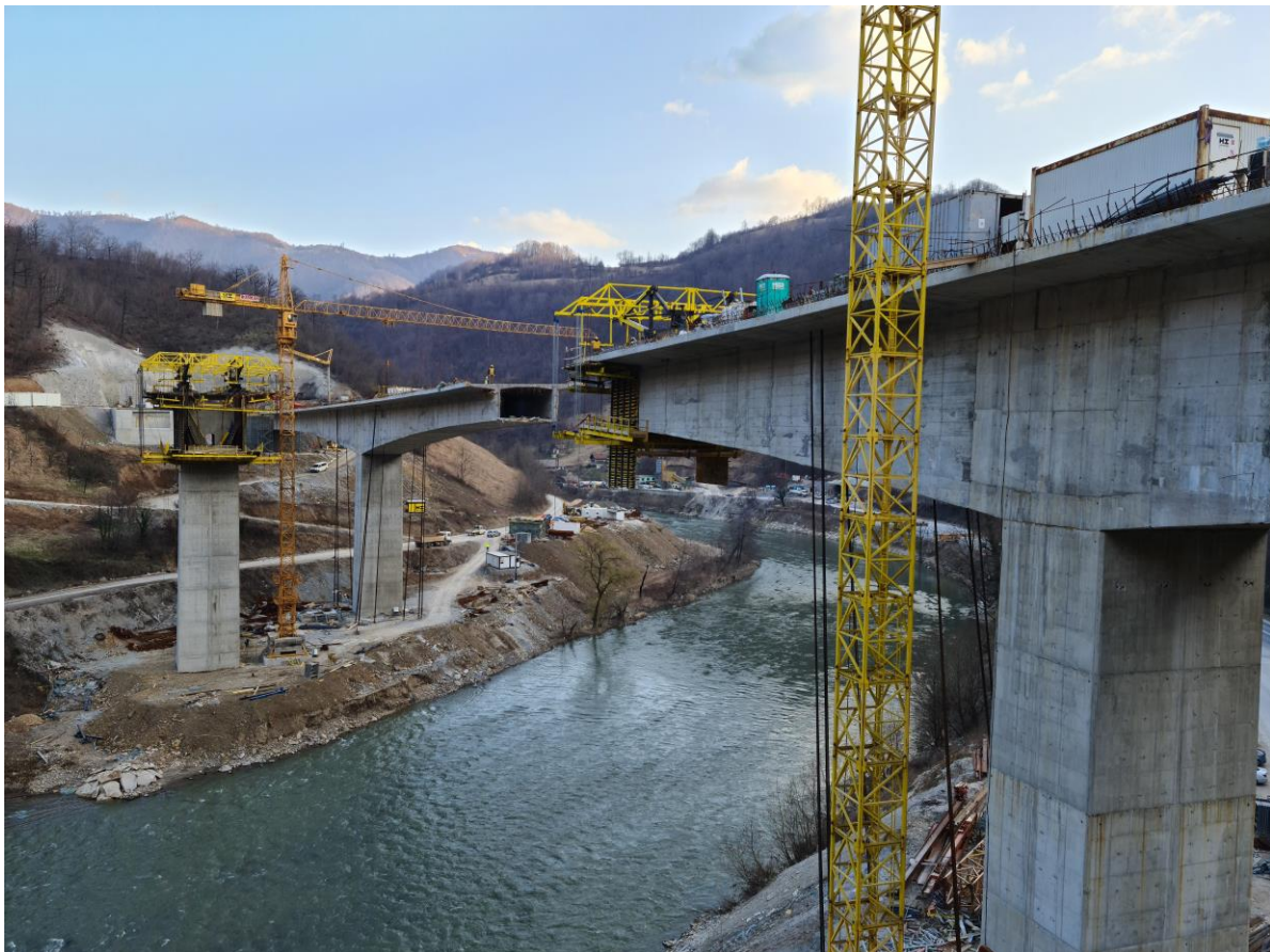
Figure 37. Vranduk 2 bridge under construction
