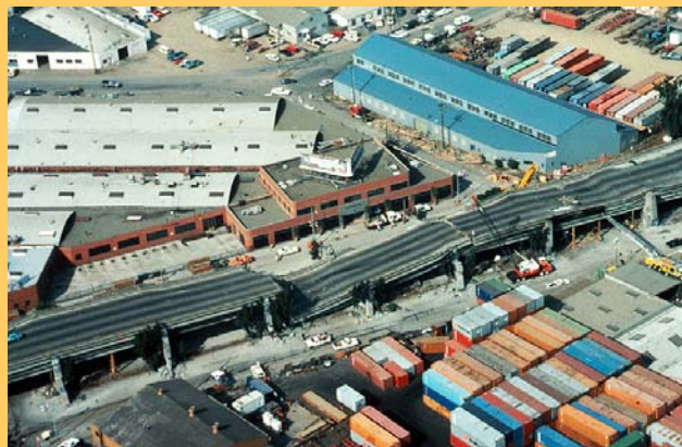
Cypress Street Viaduct, Oakland, California United States Srušio se tokom potresa, 1989. 42 poginula.
